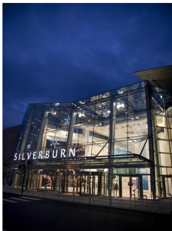
Hammerson acquired a 50% stake in the Silverburn shopping centre, Glasgow, Scotland
